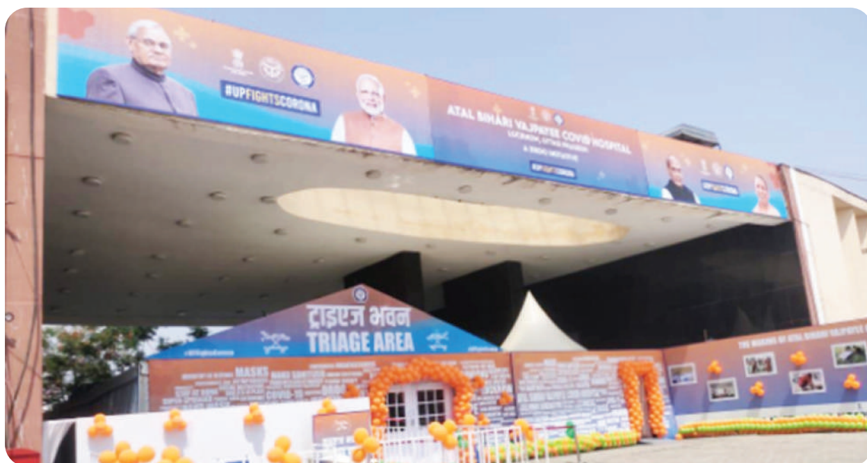
Main Entrance of Atal Bihari Vajpayee COVID Care Hospital, Lucknow, Uttar Pradesh
